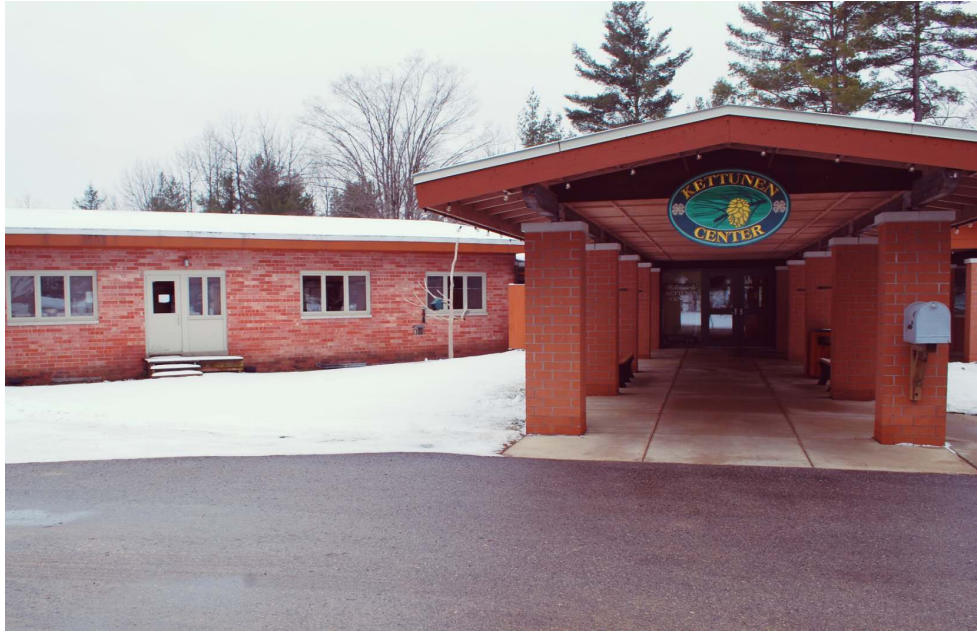
Figure: 15 Main entrance of The Kettunen Center
